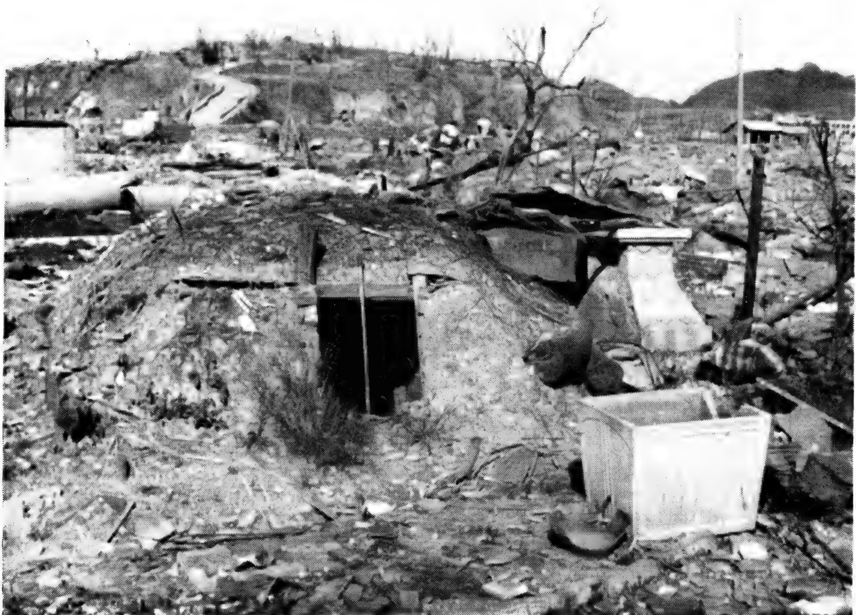
Photo No. 18. NAGASAKI. Typical small earth-covered back yard shelter with crude wooden frame, less than 100 yds. from the centre of damage, which is to the right. There was a large number of such shelters, but whereas nearly all those as close as this one had their roofs forced in, only half were damaged at 300 yds., and practically none at half a mile from the centre of damage. See paragraph 41.
